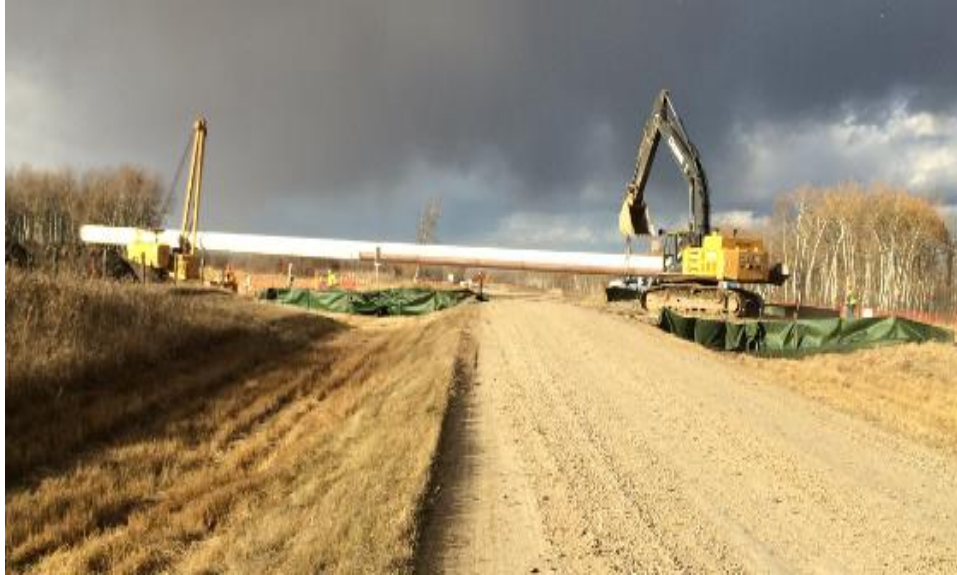
Piping crossing SF road 112
