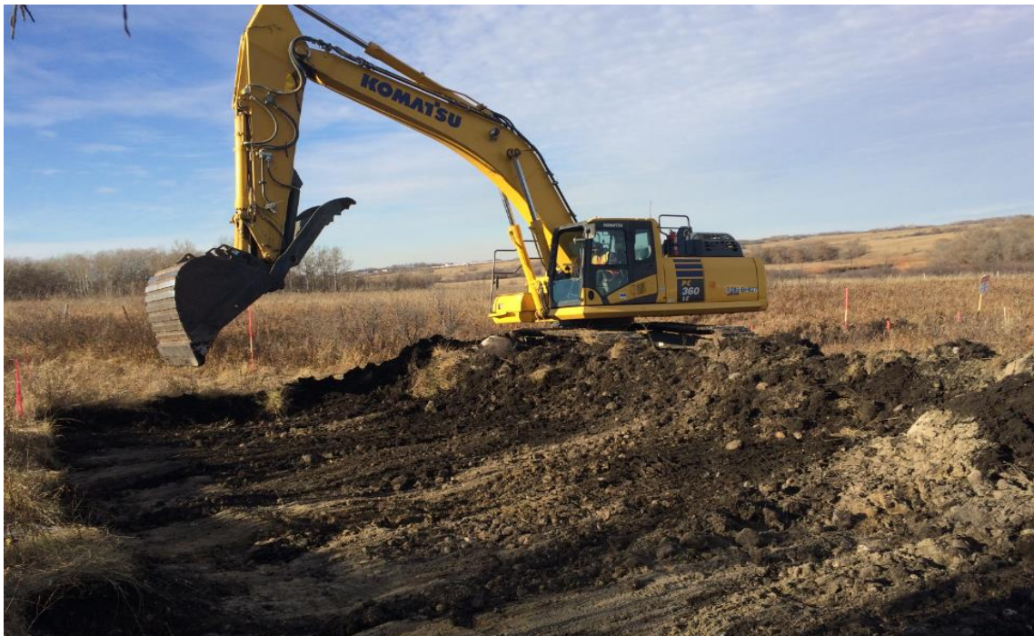
Pipestone Creek Track hoe stripping soil
