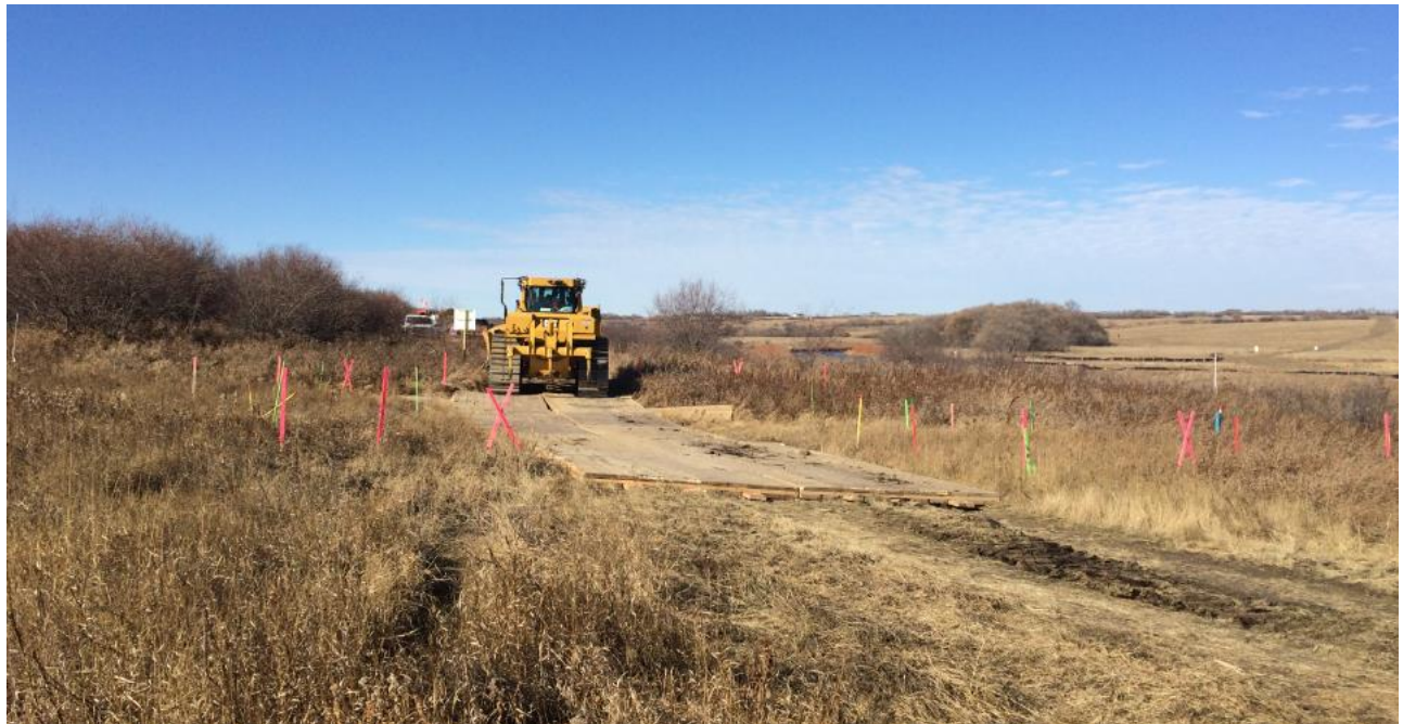
Track hoe travelling on ramp at Pipestone Creek
