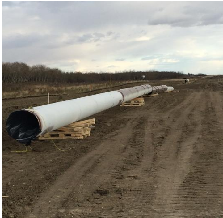
SF 113 East ROW entry Piping set on skids
