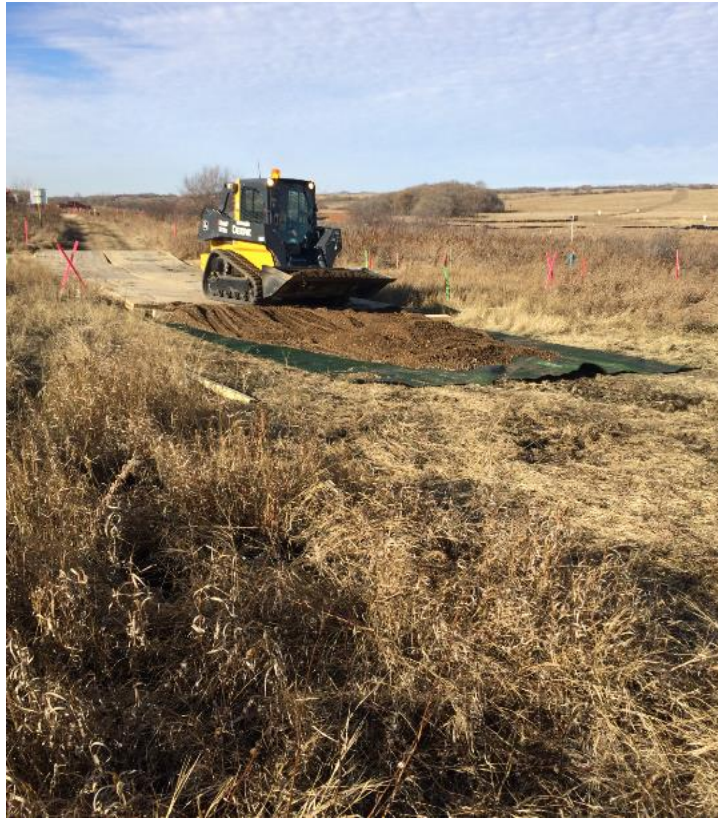
Pipestone Creek ramping underground lines
