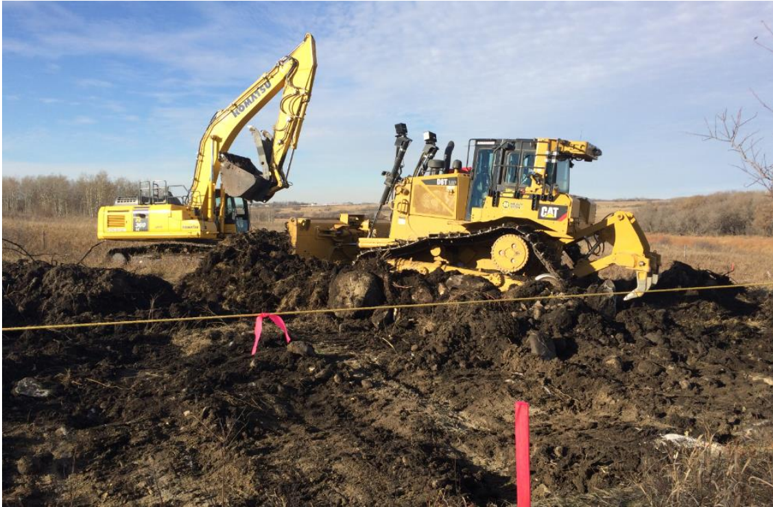
805 + 567 D6 Dozer and Track hoe
