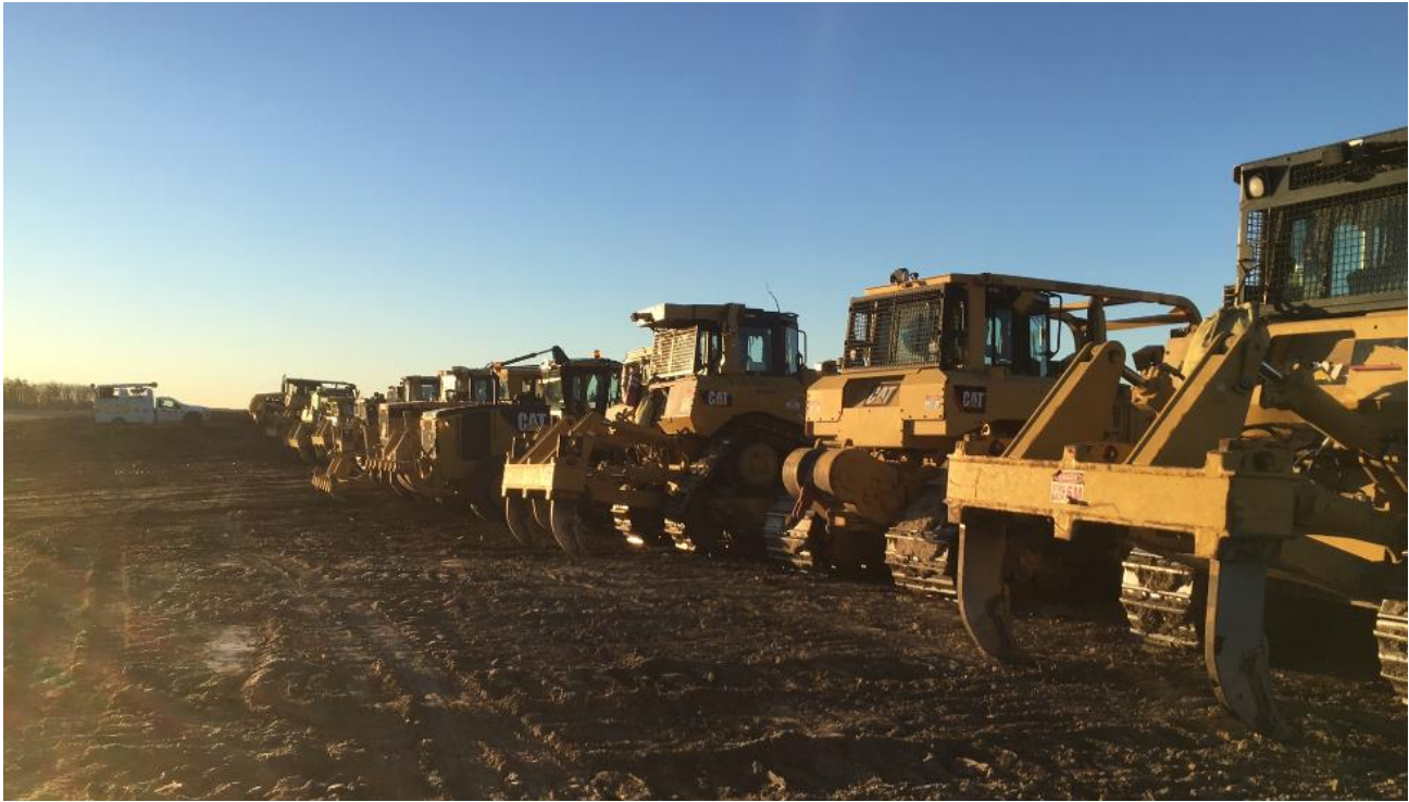
Equipment lined up at 764 + 542
