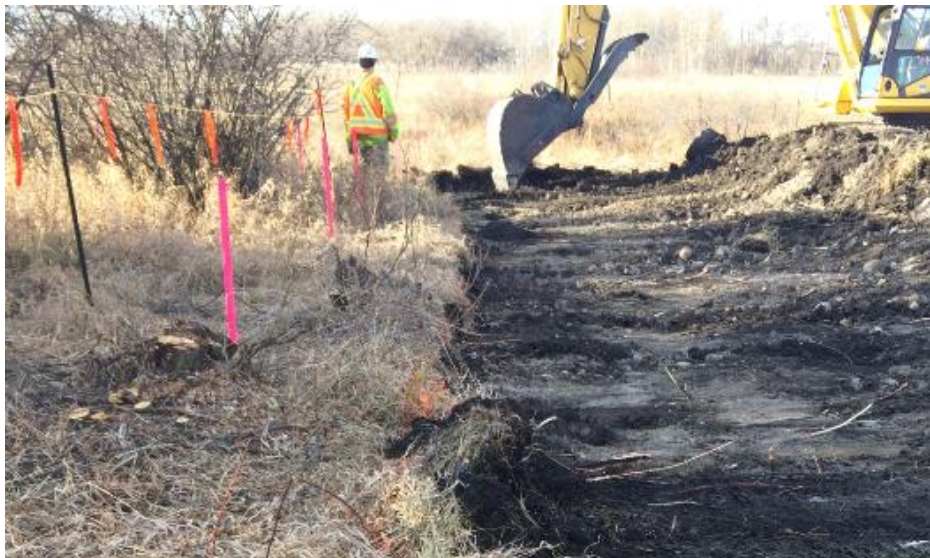
Spotting Track hoe at 805 + 600 Pipestone Creek
